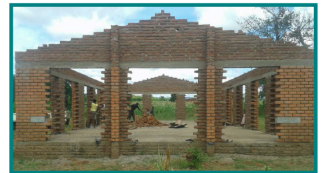
Sharon Roof Project
